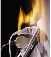
**OVERLOADED ELECTRICAL:** Homes today are brimming with state-of-the art technology, entertainment, and computer equipment. However, when too many lights and appliances are attached to the electrical system, it will overload and then overheat. The heat causes the wire insulation to melt and ignite, resulting in an electrical fire.
